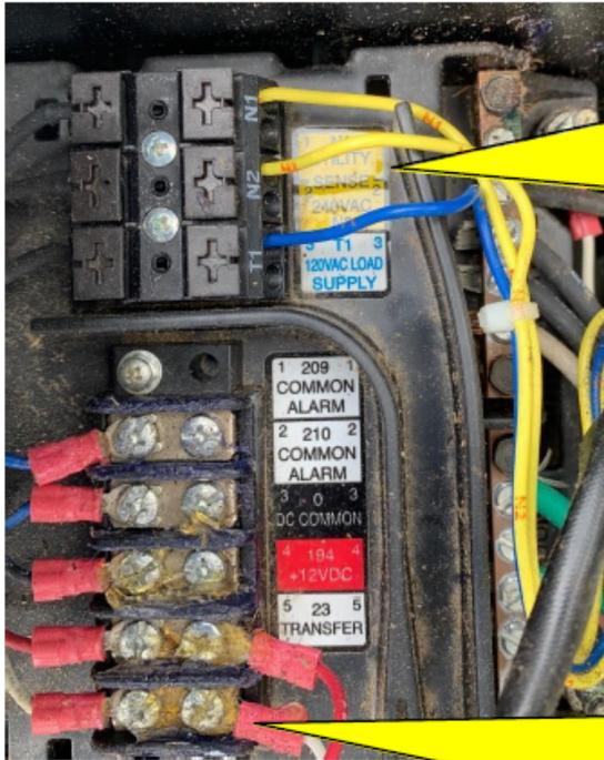
**DO NOT CONNECT THE OMNI INPUTS TO 240 VAC!!!**
