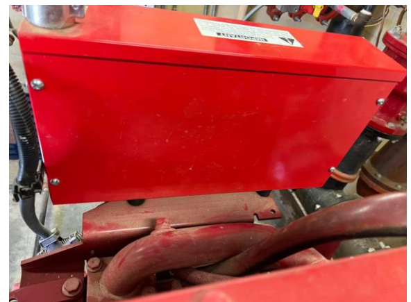
Back of Clarke Fire Control
