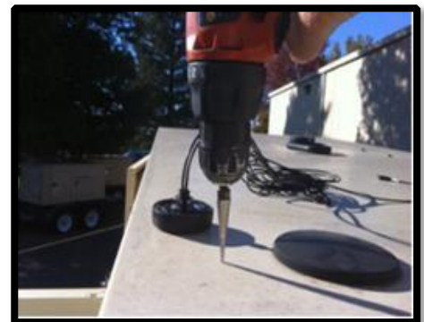
Drill ½” hole for antenna & cable
